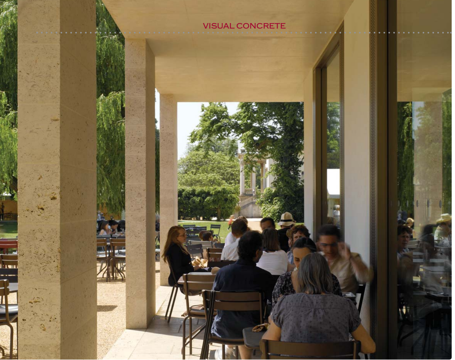
Above: View of loggia with exposed concrete soffit.
